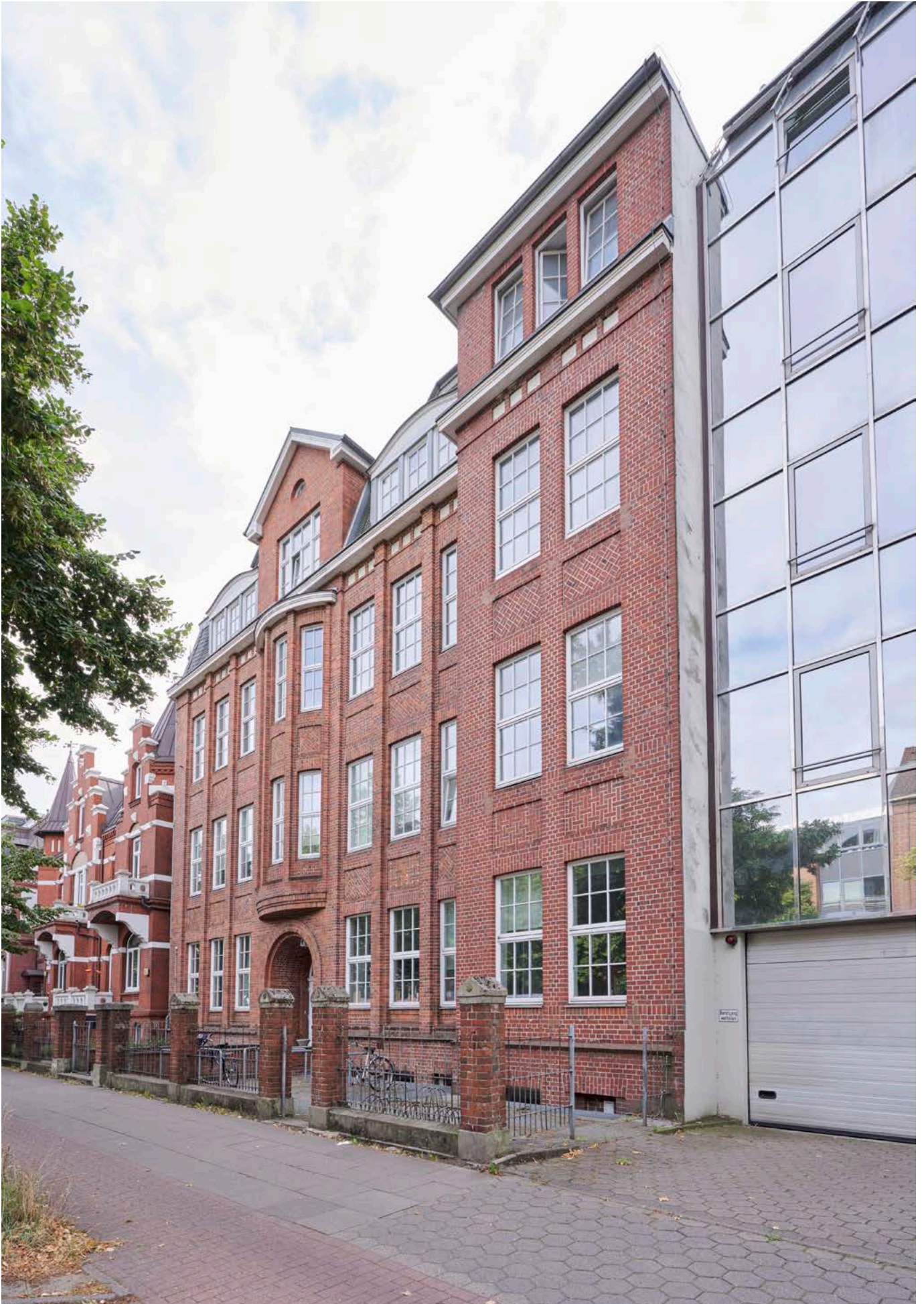
Entrance building Wartenau 15
