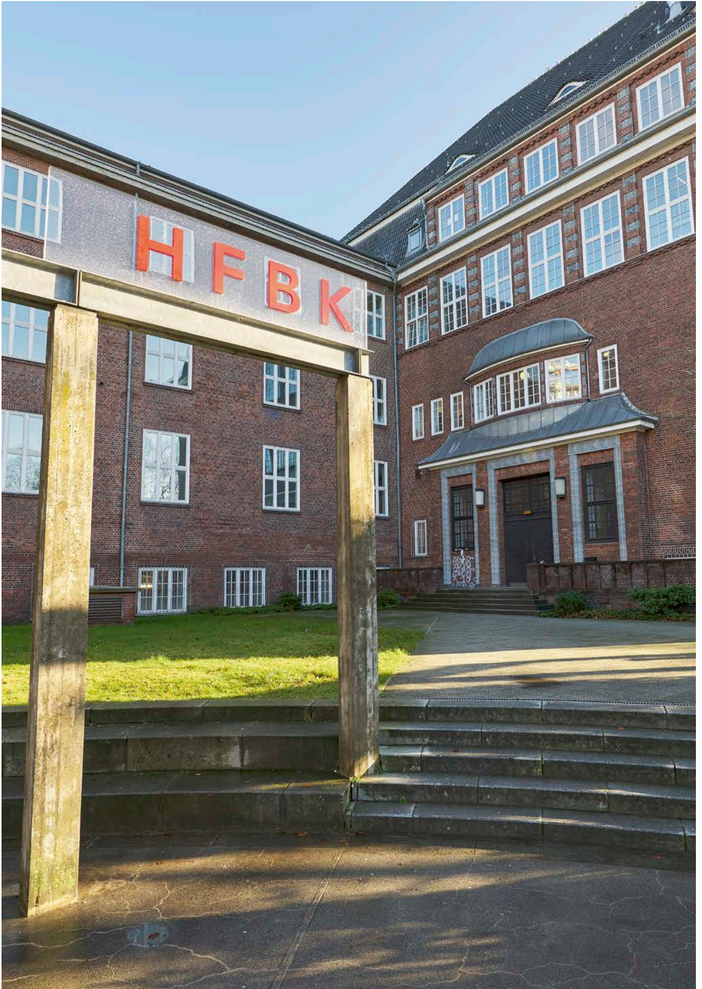
Entrance building Lerchenfeld 2
