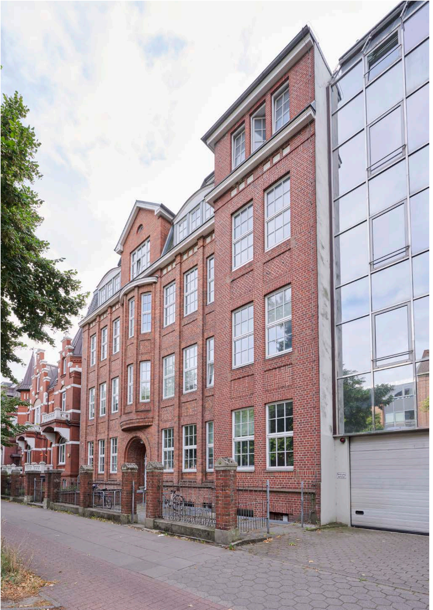
Entrance building Wartenau 15
