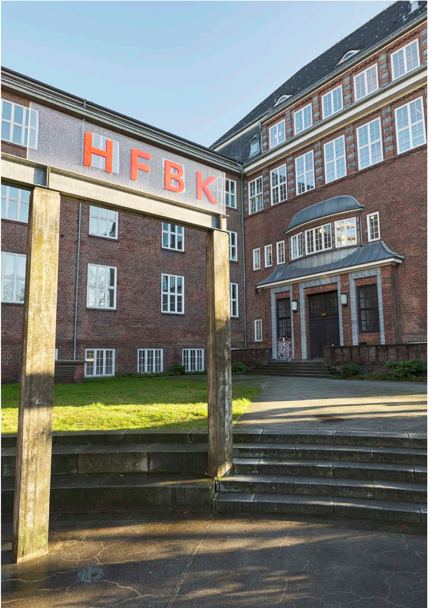
Entrance building Lerchenfeld 2
